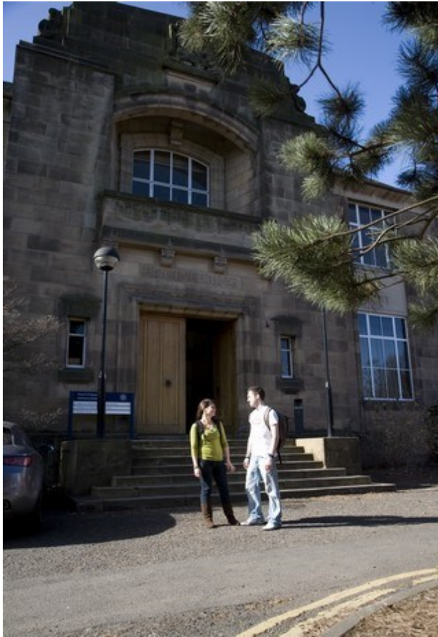
Figure 1.7 Sanderson Building at The University of Edinburgh
