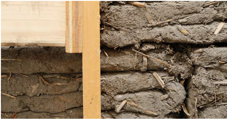
Previous. Edinburgh Eco-Pavilion. View of Pavilion. Left. Prefabricated Raw Earth Modules. Close-Up Image. Above. Additive Manual Printing of Blocks. Construction off Site. Middle. Wall Installation. Construction on Site. Bottom. Timber to Earth. Connection Detail.
