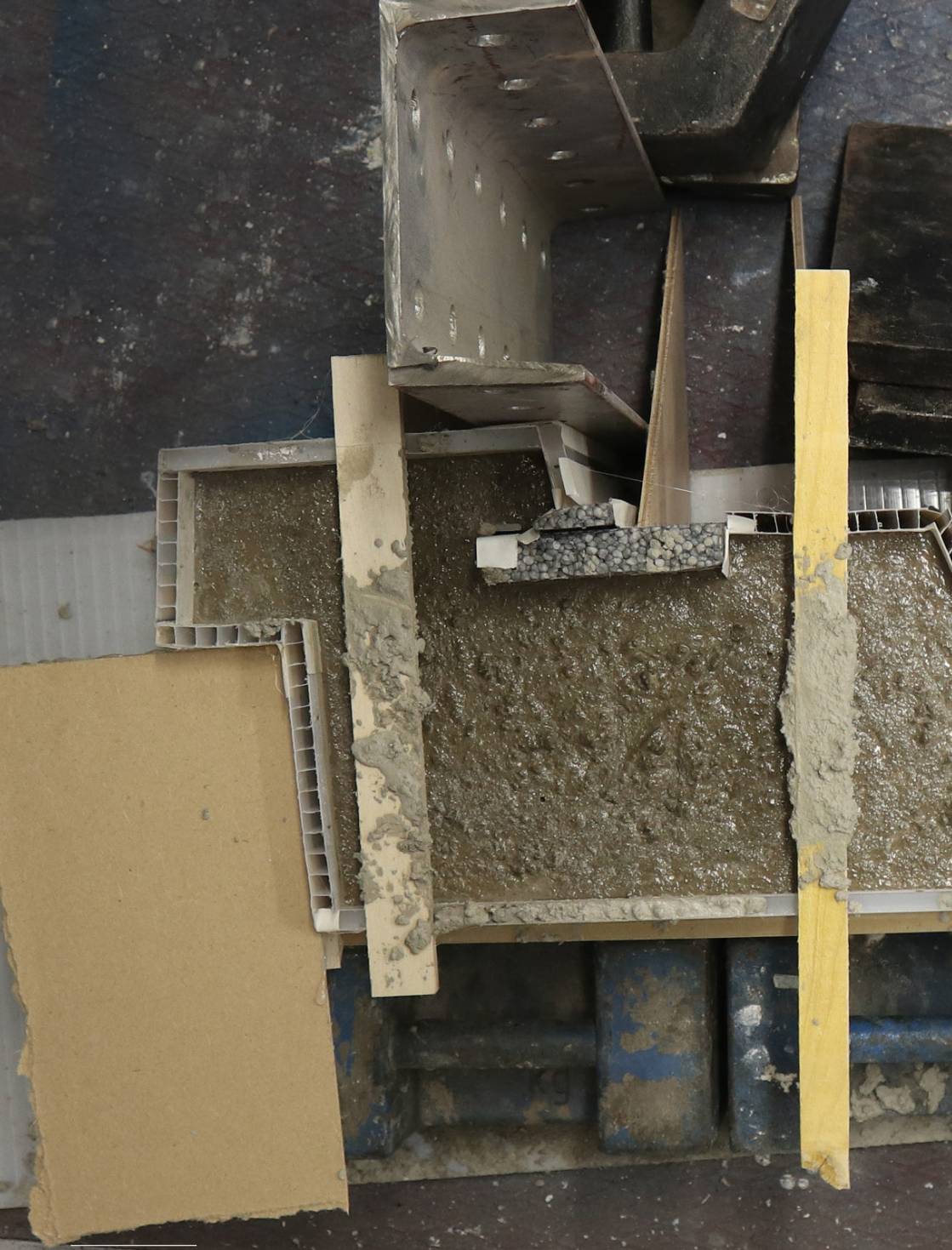
Above. Support Structure for The Ornamental Downpipe Construction Process.
