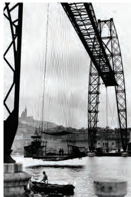
18. Transporter Bridge in Marseille 1906-1944. Image © Hulton-Deutsch Collection/CORBIS
