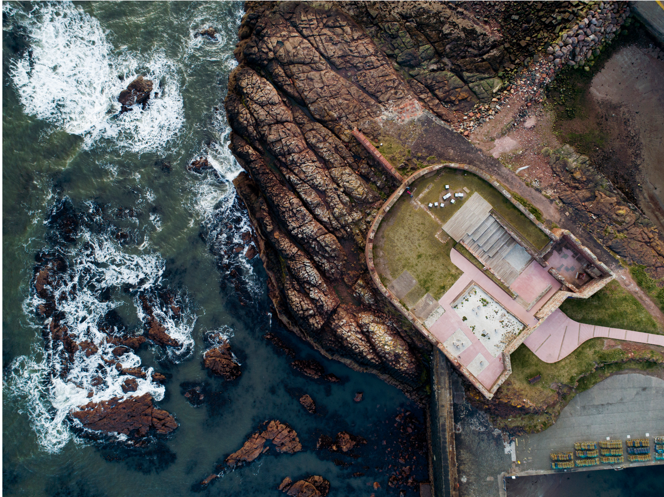
FIG. 15 Aerial view. Photo courtesy of Maclean Photographic.
