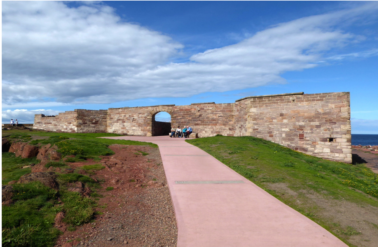
FIG. 7 View of the new access path leading to the battery. Photo Rankinfraser Landscape Architecture.
