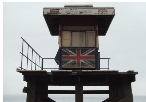
FIG. 12 End of the Pier Show
