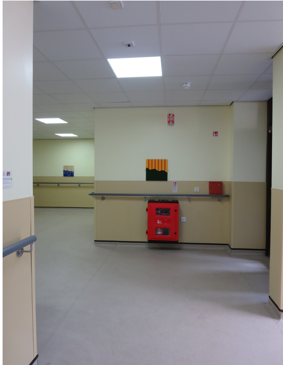
FIGS. 8-9 Hand sketches with indicative colours were used in the early consultations with users and placed in the ward. After discussion, the terracotta was changed to a stronger red. The corridor prior to the installation lacked differentiation, all walls were pale yellow. Image and photo Fiona McLachlan.
