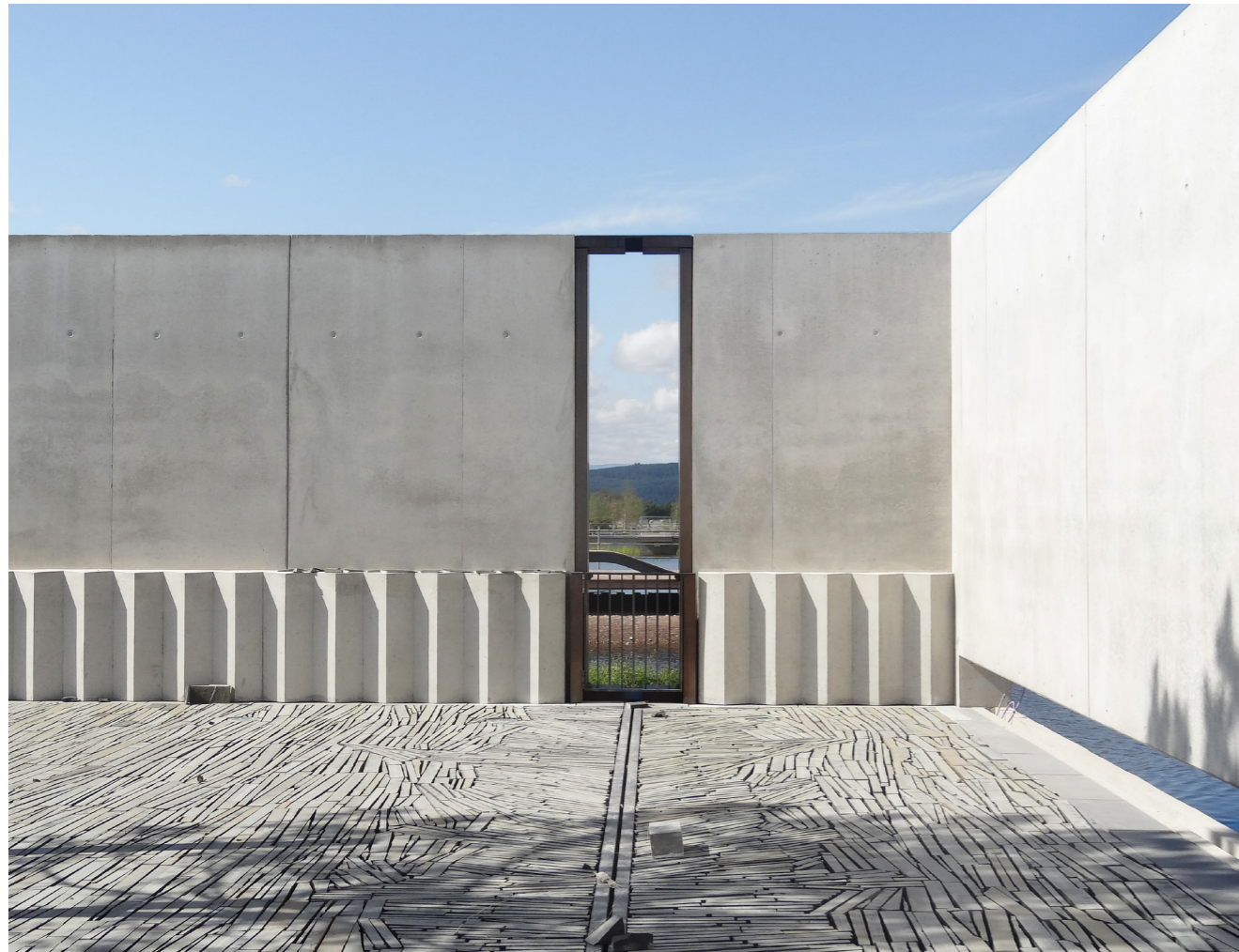
FIG. 14 The Island Gallery under construction in 2014, showing the concrete 'pleating' on the north wall and the splintered Caithness stone floor under construction. Photo Lisa Mackenzie.
