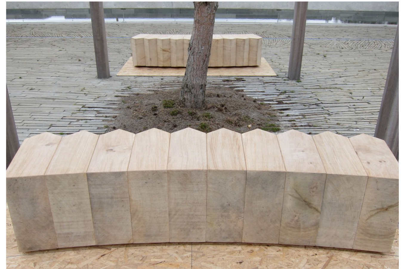
FIG. 29 The pleated timber benches were constructed from solid oak and pick up on the dimensions of the concrete pleating on the north wall. Photo courtesy of Dougal Black.
